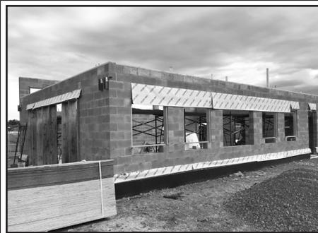
*Outdoor classroom concrete foundation and exterior block walls are complete.*
